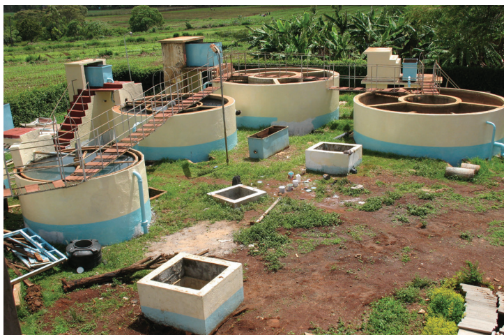
Fig. 1.5 A Water Treatment Plant in Rwanda
